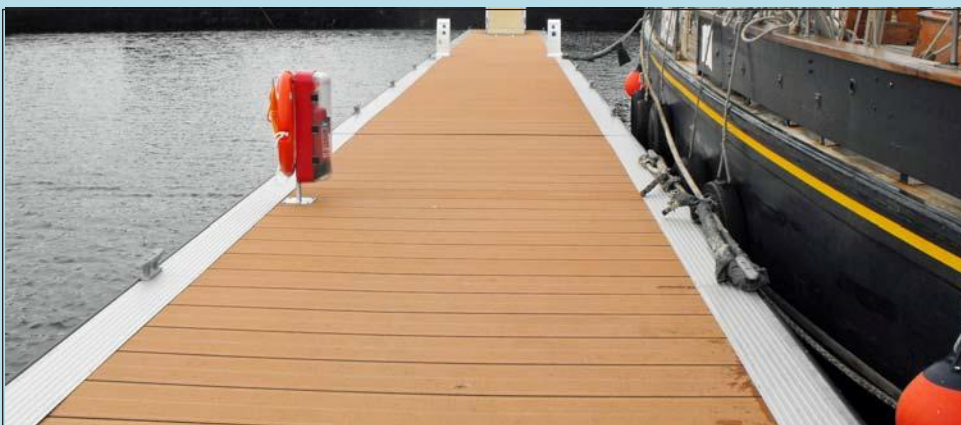
Decking grooves create anti-slip qualities
